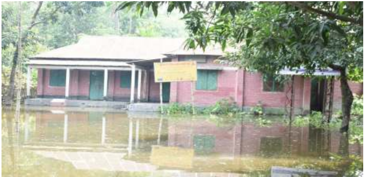
An NGO office in flood-prone area of Moghulbasha
